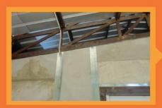
The roof is made of alu-zinc sheet modules (more resistant than the common zinc sheets), which are supported by a structure of collapsible brackets, beams and columns that hold up the roof.
