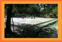
The floor-base is the reinforced concrete foundation on top of which the modular shelter is assembled.
